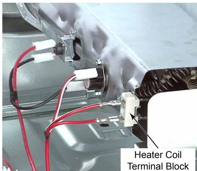
For US models: The heater element on electric dryers is designed to provide 5600 watts when operated on 240 volts.
