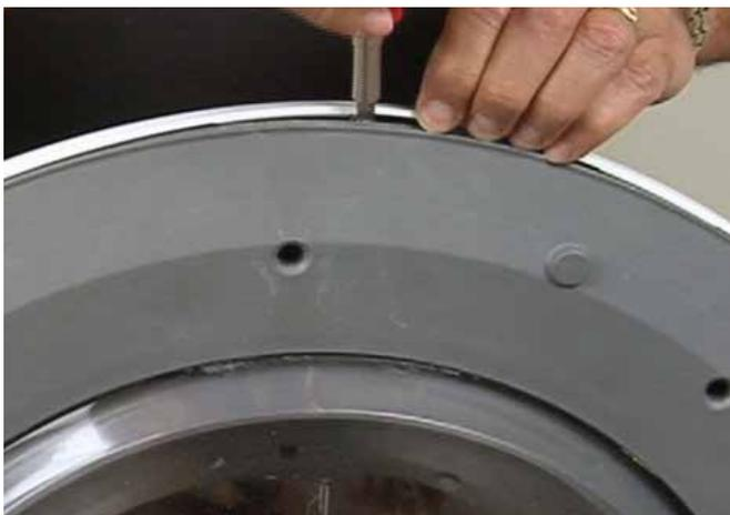
4. Use a small flat blade screwdriver to release the clips around the edge of the outer door trim to start separating it from the inner door.
